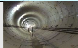
Delhi Mass Transport System Project , Subway Tunnel
