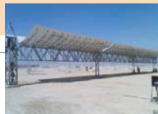
▲Planned construction site (Photo:JICA)
