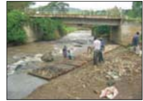
Construction of bank protection works
