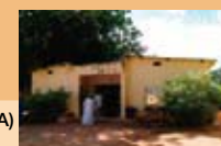
Existing health centre (new one is under construction)
