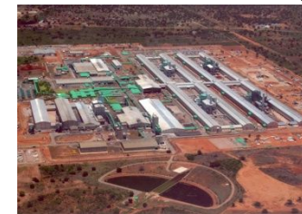
Photo: Mitsubishi Corporation
