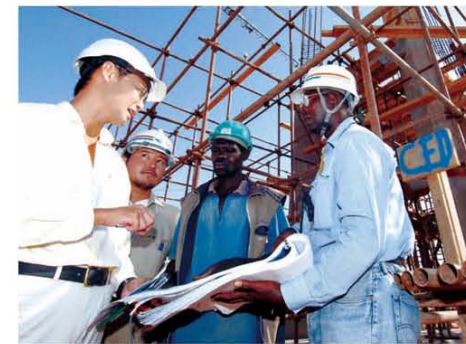
A Japanese architectural expert giving guidance on building a water tower (Senegal) Photo: JICA
