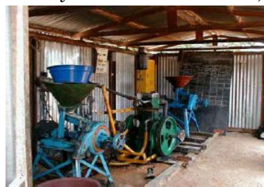
(Multi-functional diesel-based power plant system)
