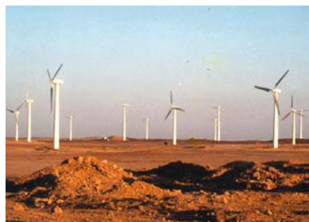
(Zafarana Wind Power Plant)
