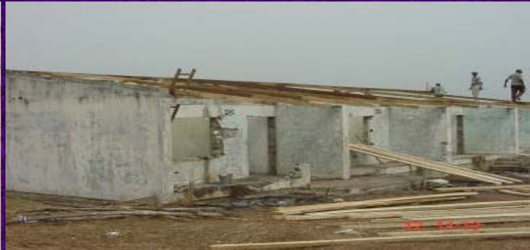
Rehabilitation works at a returnee Way Station, Liberia
