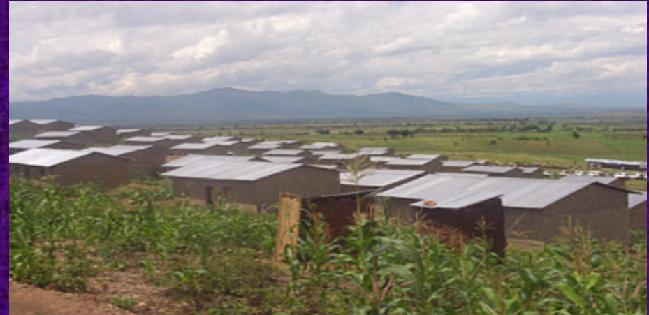
Some of the homes built for refugee returnees and other destitute people , Gatere village, Burundi
