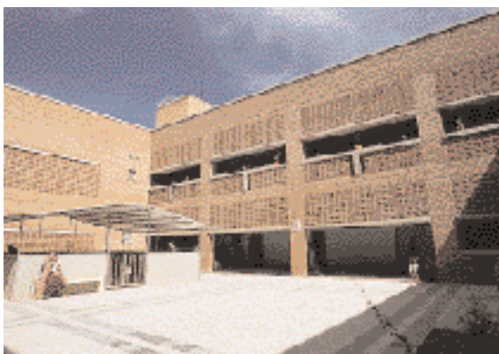
Yemen's national tuberculosis research institution, the construction of which was financed by Japanese grant aid.
