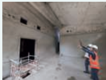
Site inspection with local engineers (the author, foreground)
