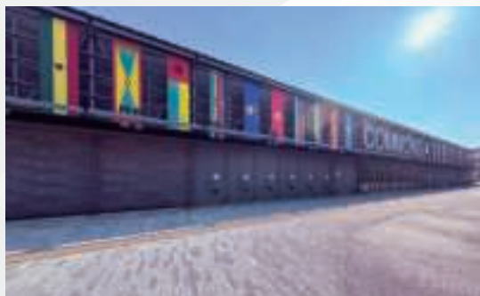
▲ Exterior view of Commons-A (Osaka; Photo: Japan Association for the 2025 World Exposition ©Expo 2025)
