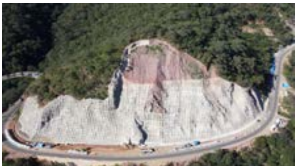
Disaster risk reduction work to prevent slope collapse and mudslides along the road under the “The Project for Road Disaster Prevention of National Road No. 7” grant aid for Bolivia (June, Santa Cruz Department, Bolivia)
