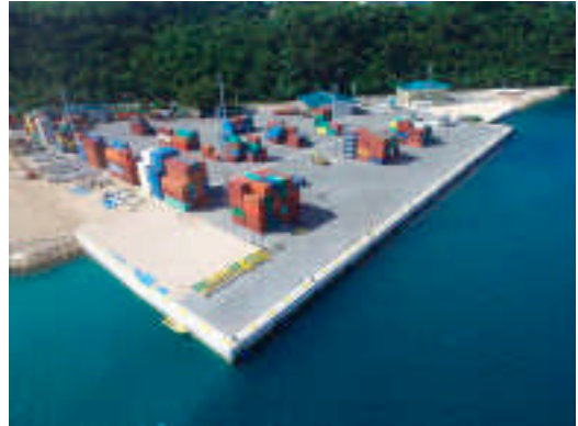
Port Vila Lapetasi International Wharf constructed with assistance from Japan (Vanuatu)
