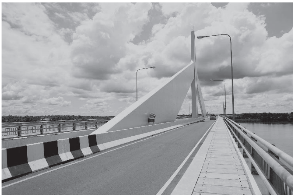
The Second Mekong International Bridge, constructed through an ODA Loan (Second Mekong International Bridge Construction Project), connects Thailand and Laos, spanning a distance of approximately 1,600 m (Photo: Yasuhiko Okuno / JICA)
