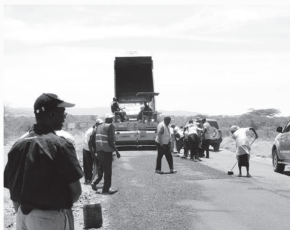
Pavement resurfacing work takes place along a road through savanna. (Photo: Motohiko Nishibayashi)
