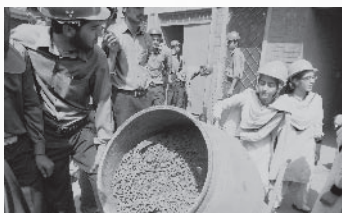
Students learn how to work with concrete (Photo: Minoru Ito)
