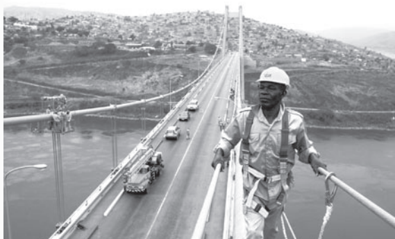
OEBK workers maintain Matadi Bridge (Photo: Shinichi Kuno / JICA)
