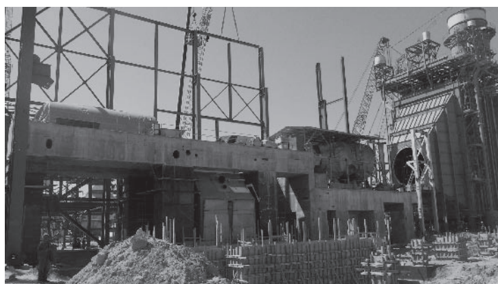
Shimal gas combined-cycle power plant in Azerbaijan (second unit construction project).
