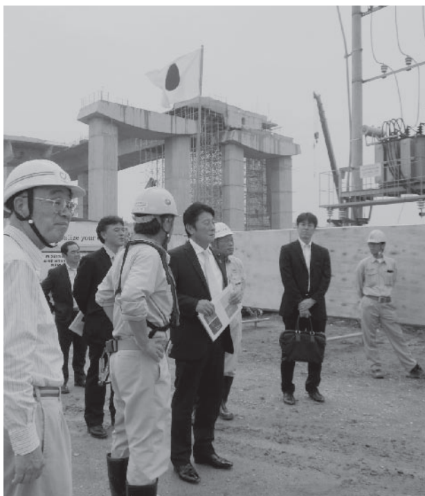
Former Parliamentary Senior Vice-Minister for Foreign Affairs Masaji Matsuyama visiting the construction site of the Nhat Tan Bridge in Viet Nam.
