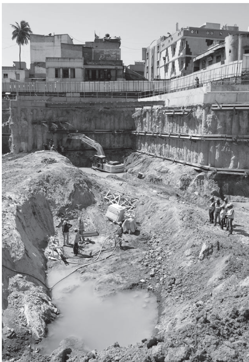
Construction site of metro in Bangalore, India. Excavation work at the Chickpete Station, where the density of building is high. (Photo: Shuhei Fujita)
