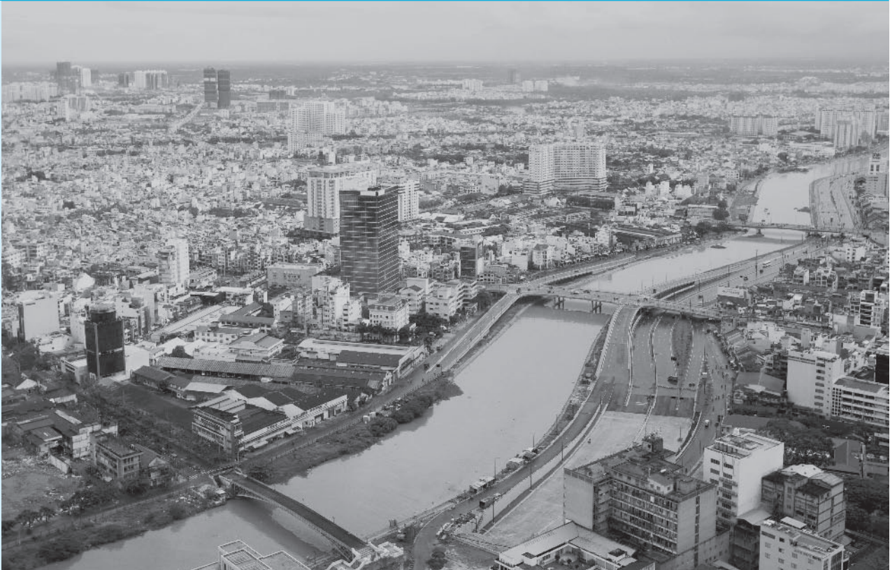
Ho Chi Minh City overlooking the Saigon East-West highway tunnel under construction in Viet Nam (Photo: Hikaru Nagatake / JICA)
