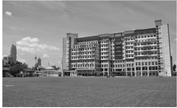
New campus building completed in February 2012. (Photo: JICA)
