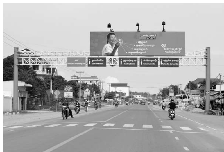
Construction is complete on the new, improved Cambodian National Route 1. (Photo: Koji Sato/JICA)
