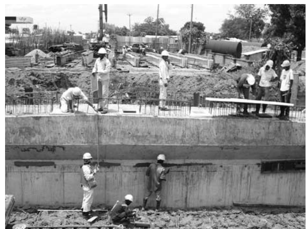
Japanese engineers work together with local workers for promoting technology transfer. (Photo: JICS)
