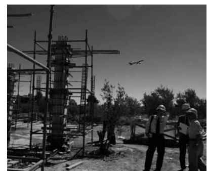
Installing an X-ray inspection system. (Photo: JICA)
