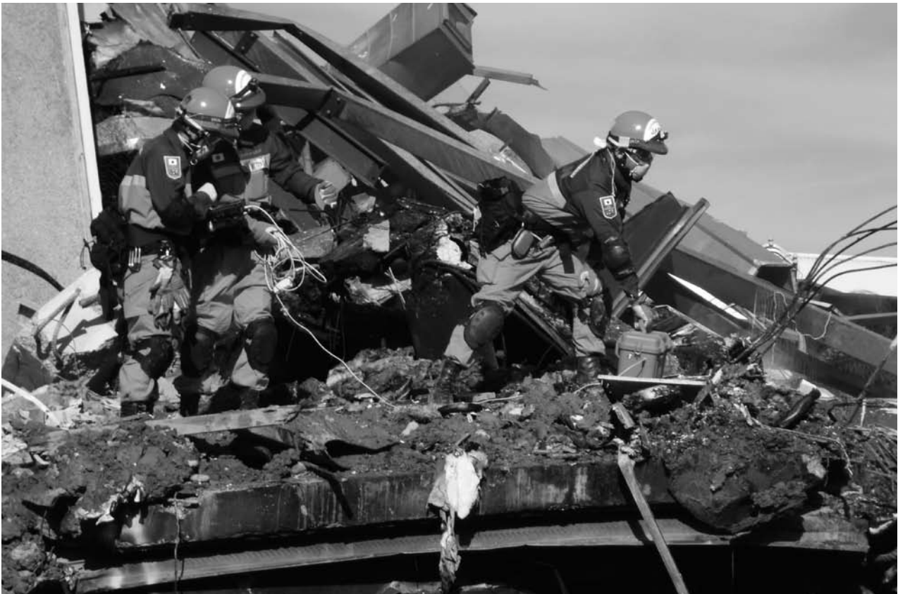
The Japan Disaster Relief Team conducts a search and rescue in an area afflicted by the New Zealand Earthquake. (Photo: JICA)
