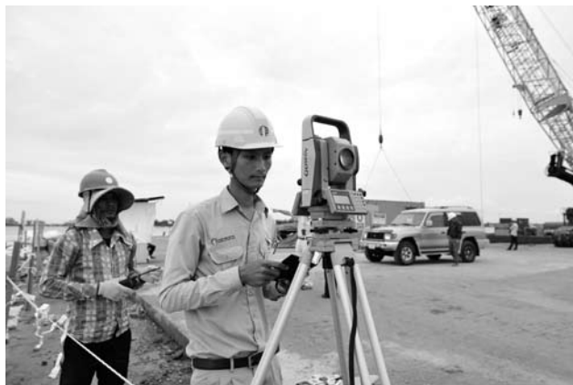
Project for Construction of Neak Loeung Bridge in Cambodia Vietnamese engineers survey the planned site for construction of the Neak Loeung Bridge. (Photo: Koji Sato/JICA)
