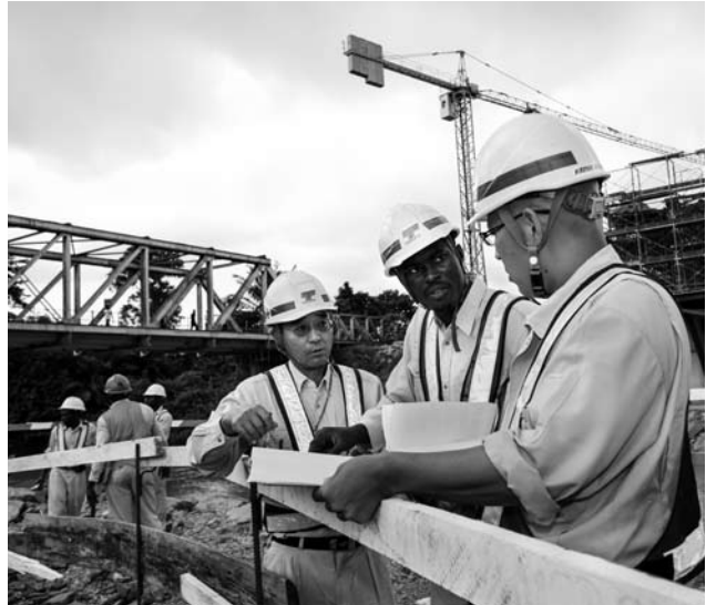
Repair work on a national road. Engineers from Japan and Ghana check progress at the site of bridge construction. (Photo: Akio Iizuka/JICA)
