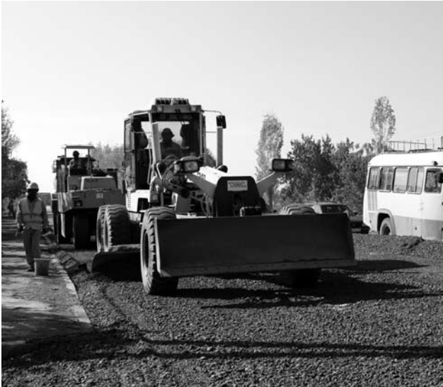
Construction site of the national road connecting the border of Afghanistan with the capital of Tajikistan. (Photo: Shinichi Kuno/JICA)
