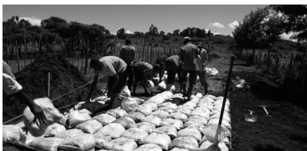
The use of CORE’s “Do-nou” construction method allows local residents to easily make repairs by themselves. (In Rift Valley Province, Kenya) (Photo: CORE)
