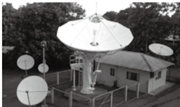
A satellite communication earth station used for the construction of a distance-learning network (USPNet) as part of the "ICT for Human Development and Human Security Project" in Fiji. Distance-learning programs are provided from this location to remote campuses and learning centers in 12 Pacific Island countries. (Photo: Kader Hiroshi Pramanik)
