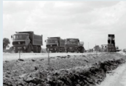
A view of construction of a road between Arusha and Namanga (Photo: East African Community)
