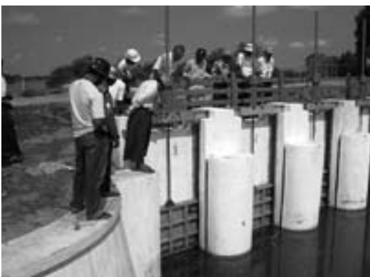
Confirming the status and function of the sluice gate after repairing the circle sluice gate as part of the "Project for Preservation of Farming Area for Urgent Rehabilitation of Agricultural Production and Rural Life in Areas Affected by Cyclone Nargis" in Myanmar (Photo: JICA)
