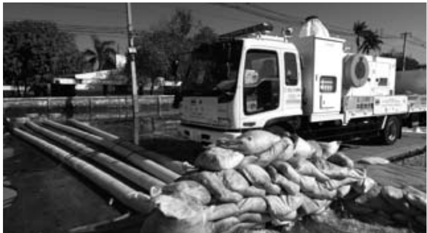
Japanese drain pump vehicles conduct work at industrial parks in Thailand. The drainage capacity of each truck is 30 m 3 per minute. (Photo: JICA)
