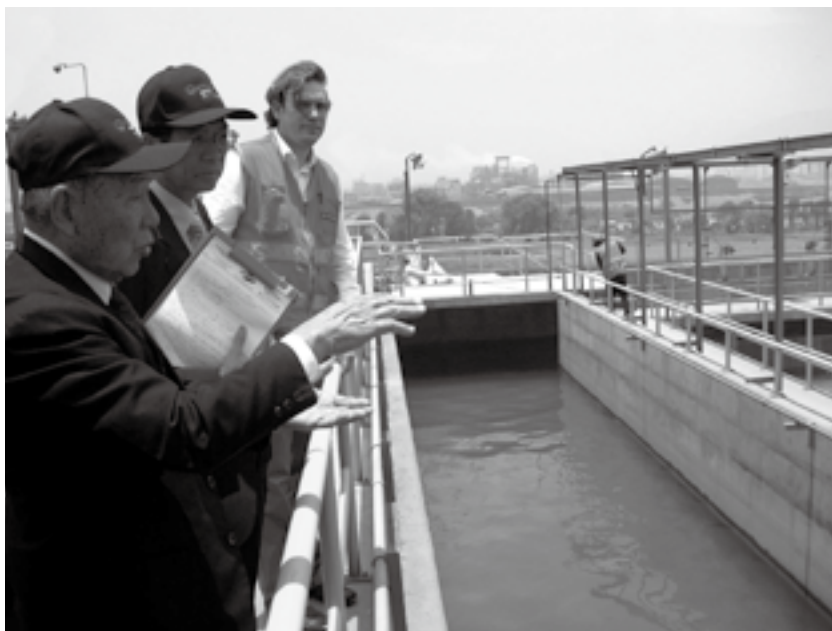
A Japanese evaluation team inspects the site of the "North Lima Metropolitan Area Water Supply and Sewerage Optimization Project" that Japan implemented in Peru
