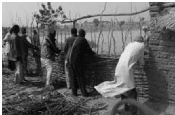
The “Support to the Improvement of School Management through Community Participation (School for All) Project” Members of the community in Niger repair a school on their own (Photo: Hiroyuki Uemura)
