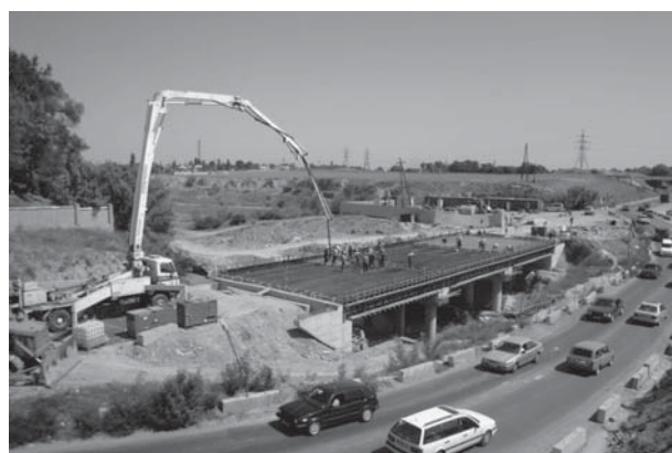
Construction work for the floor slab of the Alamedin bridge under construction (Kyrgyzstan) (Photo: JICA)
