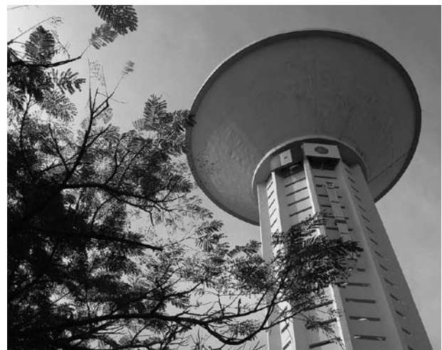
Water tower in Senegal (Photo: Kenshiro Imamura/JICA)
