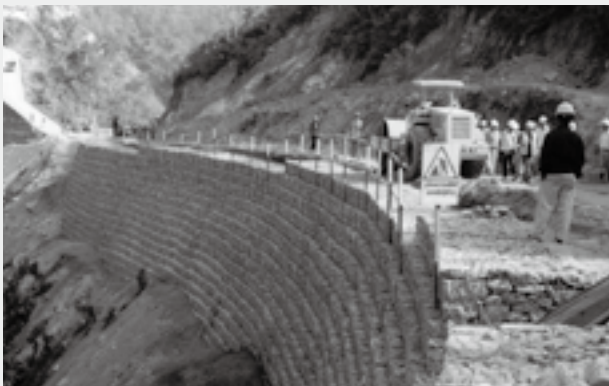
Stone wall utilizing local materials. (Photo: Nippon Koei Co., Ltd.)
