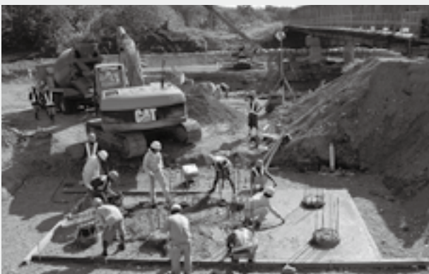
Workers carrying out construction of a foundation. (Photo: Mr. Nakano)
