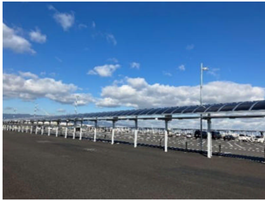
Perovskite solar cells installed at EXPO, Osaka-Kansai Transportation Terminal(Photo: Ministry of Economy, Trade and Industry)
