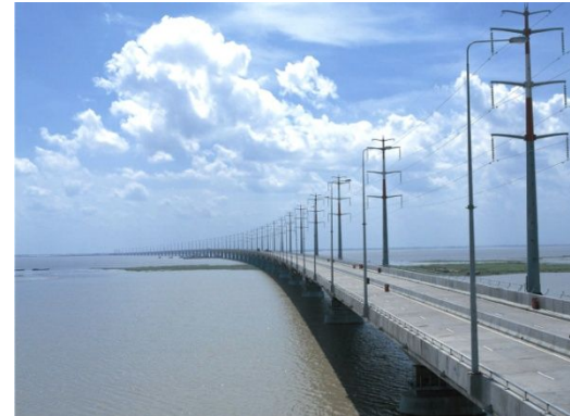
(Jamuna Multipurpose Bridge, The western part of Bangladesh)
