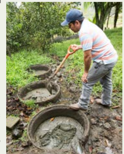
▶ Creation of a biogas plant using receiving tanks (Costa Rica: Project for Promoting Participatory Biodiversity Conservation) Photo provided by Kenshiro Imamura/JICA
