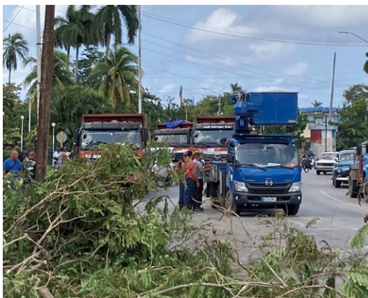
Disaster restoration work after Hurricane Ian
