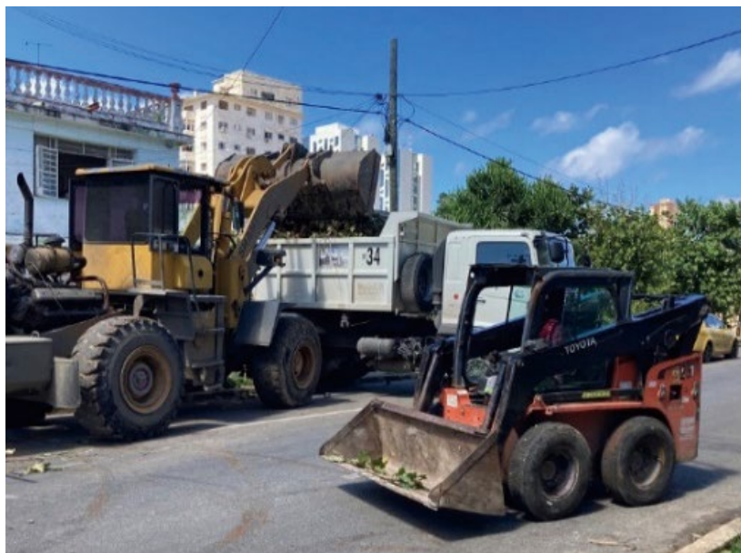
Disaster waste removal in progress: Dump truck and skid steer loader
