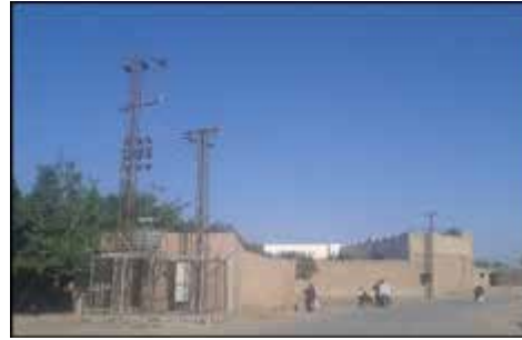
Electric transmission facility constructed by "Local Development Project" in Afghanistan (External evaluation)
