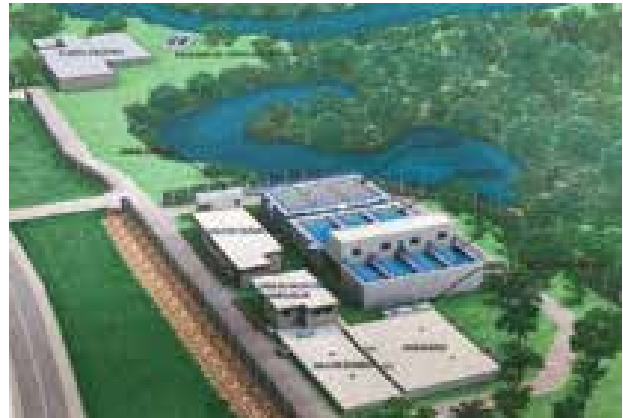
Water supply facility for Coronel Oviedo City visited in field survey (rendering)
