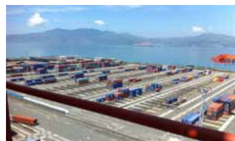
View of container terminal of "Subic Seaport Development Project" in Philippines (Deepening sector issue)
