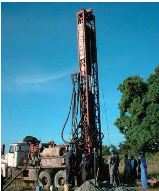
Water supply planning in region near capital (Phase 2: image of digging for test well)
