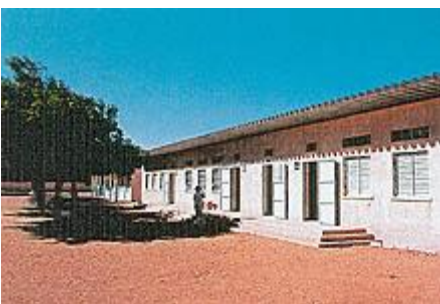
Primary school built with Japanese grant aid (near Dhakar, Senegal)
