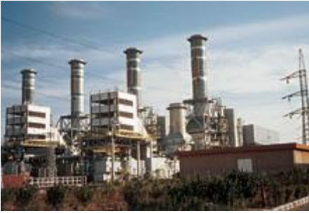
Jandar Thermal Power Station Construction Project: generating facilities
