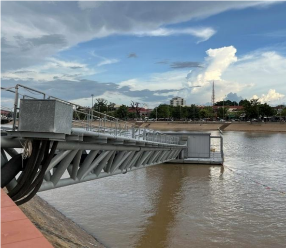
Left photo: The Sen River, a source of raw water, and the intake facility (Source: Photographed by the evaluation team during the Field Survey)
