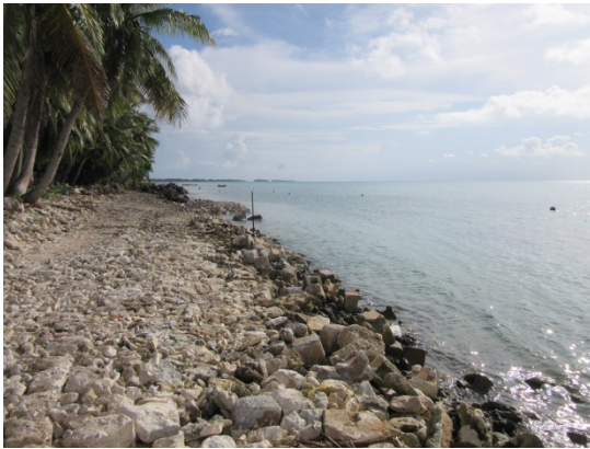
Shingle beach developed for coastal disaster measures, at the pilot project site (Tuvalu)
