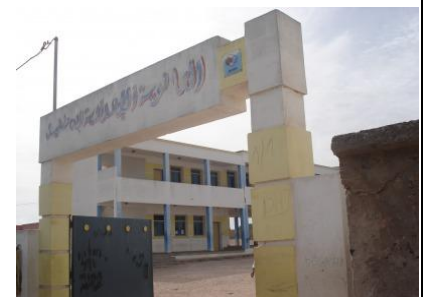
A Middle School Constructed in El Jadida Province (Photo: Evaluation Team)
