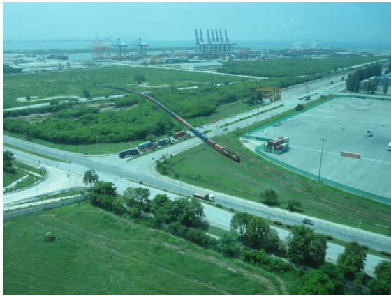
Laem Chabang Industrial Estate (Thailand)
