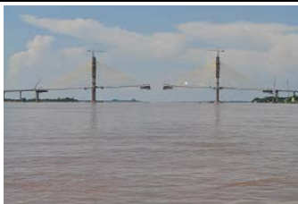
The Project for Construction of Neak Loeung Bridge (Cambodia)
