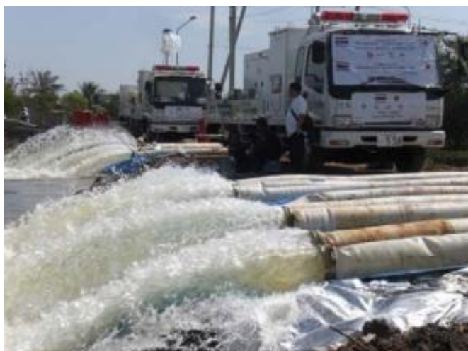
Figure 8: Drainage work (Flooding in Thailand, November 2011)
