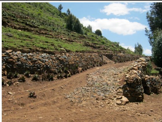
Ethiopia: Stone wall to prevent soil erosion constructed under WFP's MERET (Managing Environmental Resources to Enable Transition to More Sustainable Livelihoods) Project (Kusaye, Girar Jarso Woreda , Oromia Region)
