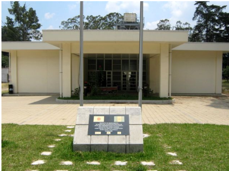
TB Specialized Hospital (Grant Aid) (The plate shows that this hospital was built with Japan's ODA)
