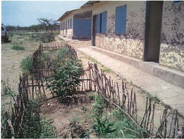
Classroom blocks and flower beds constructed by the community members supported by the ManaBU Project, Ethiopia
