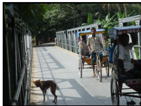
Portable steel bridge in Sadar Upazila, Faridpur
